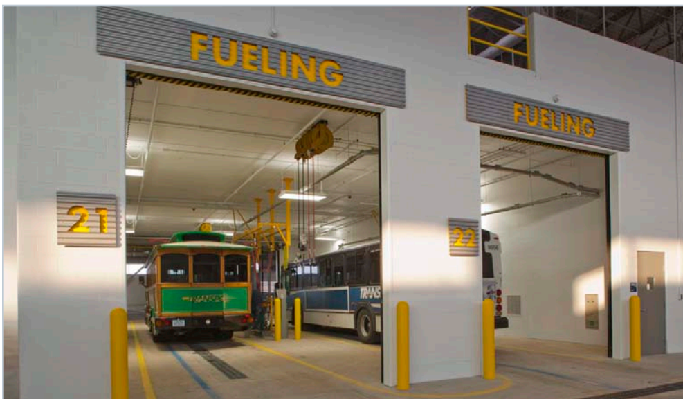
Interior Fueling Island
